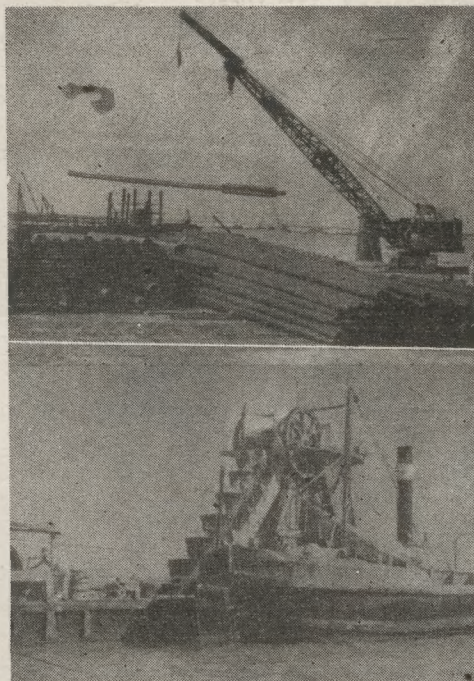
Above, left, is shown the submarine pipe bank nearly completed for launching. The horizontal portion will be buried under the floor of the harbor in a trench dredged across the west entrance channel, and ships will pass through the 500-foot space between the "risers". Right, at top, hundreds of tons of material are being transported to the site on barges. Being swung aboard is a pile with "lags", or bolted-on cleats that increase the resistance of the pile. Below, the bucket dredge chews out a trench on the harbor floor for the pipelines.
